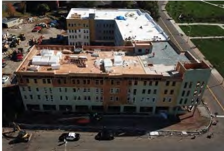
New Elevated Construction
