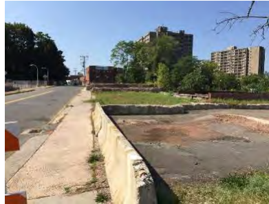
Removal of Structures from Floodplain
